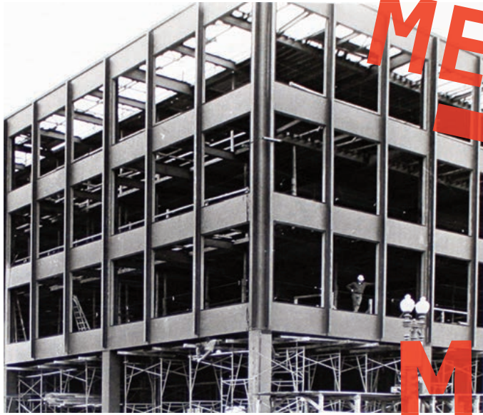
MLK Jr. Memorial Library under construction 1968-1972
